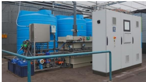
Figure 3-10. An example of a pilot installation for electrophysical precipitation in a horticultural greenhouse
