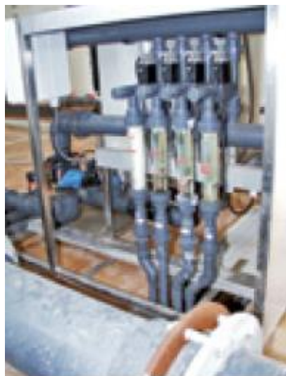
Figure 8-10. Installation of Venturi injectors inserted in a linear collector (Source: J. Antonio Marhuenda)
