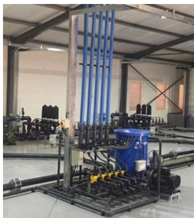
Figure 8-13. Picture of automatic fertigation equipment with mixing tank and vertical pipes ( https://pbs.twimg.com/media/DFIXyzUUQAEiEL.jpg )
