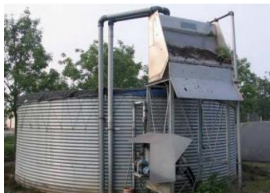
Figure 6-17. Picture of a slow sand filter (Belgium) with a sieve bend to get rid of coarse organic material before disinfecting it with the slow sand filter
