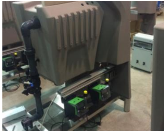
Figure 8-14. Picture of automatic fertigation equipment with mixing tank and membrane pumps (Source: J. Antonio Marhuenda)
