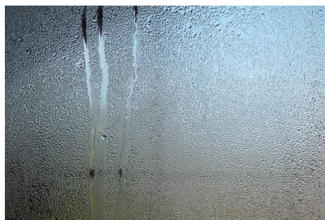
Figure 2-35. Condensation on a greenhouse glass wall
