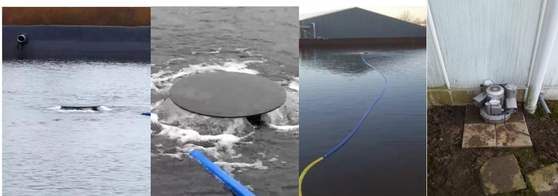
Figure 6-20. Airlift installation
