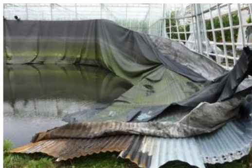
Figure 2-9. A silo has cracked due to corrosion of the lower plates ( http://www.hyente.com/nieuws.html )
