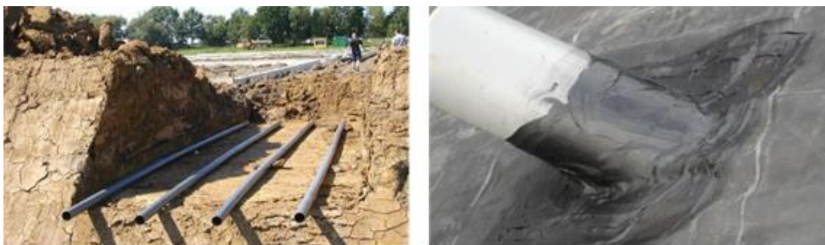
Figure 2-6. Installation of a waterproof pipeline through one of the dikes (Source: PSKW)
