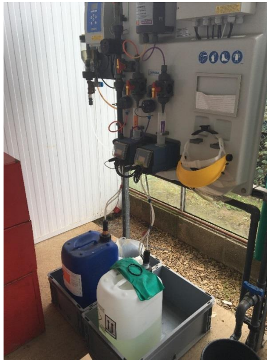
Figure 6-2. Sodium hypochlorite injection system using an electric pump and reservoir water at a UK ornamental nursery
