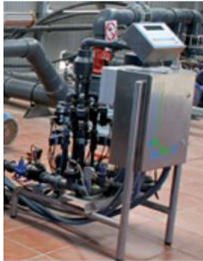
Figure 8-11. Installation of Venturi injectors in a circular configuration (Source: J. Antonio Marhuenda)
